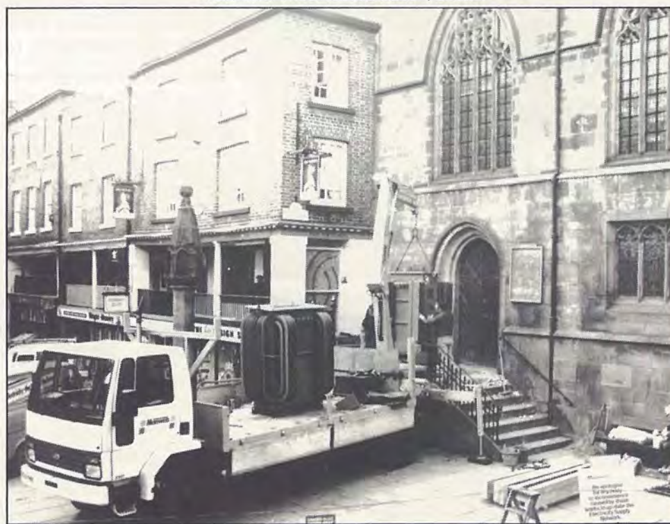
The major refurbishment of the electricity network is under way, and a new transformer is installed in The Cross sub station, Chester
